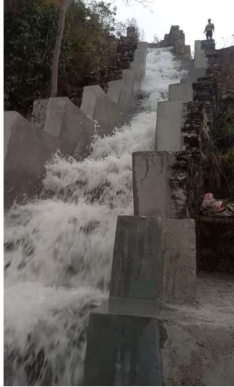
(Chute drain from Forebay Silt Extruder exit point to Anchor Block-5)
