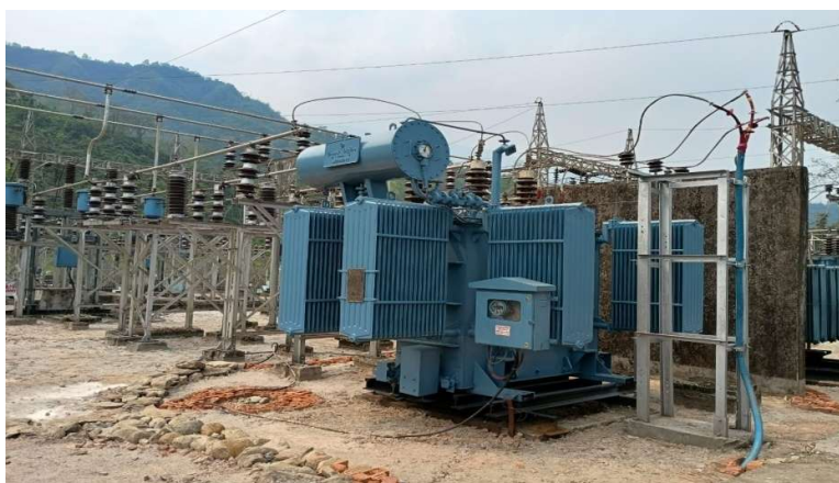
(5 MVA 11/66 Transformer at JHP –II)
