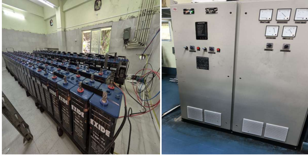
(535 Ah Battery Bank and Battery charger)
