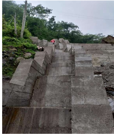
(Chute drain in front of Adit-I of LICS)
